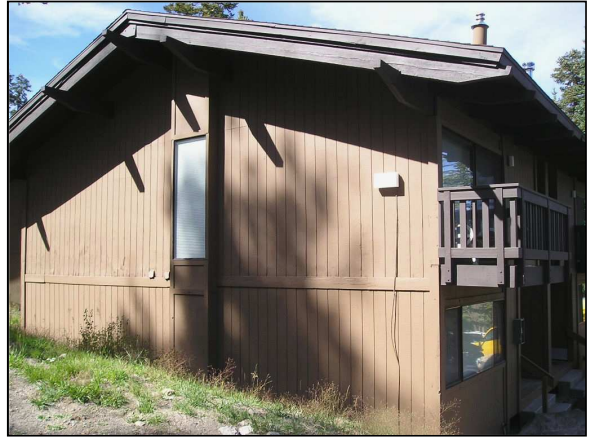
Siding & Wood Trim - Paint
