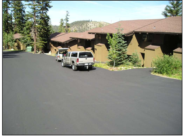
Asphalt Paving (Sealcoated in 2011)
